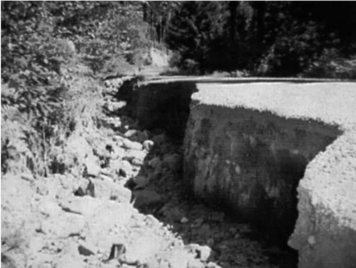
Figure 3—Severe gullying at Breitenbush flood-assessment site.
