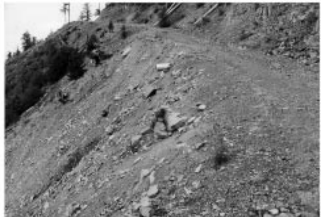
Figure 7—Initiation of debris slide at Devil's Creek flood-assessment site.
