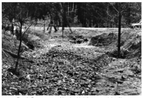
Figure 3—Terraces upstream of the culvert inlet indicate past ponded conditions. Channel dimensions and hydraulic capacity of this culvert should be checked.
