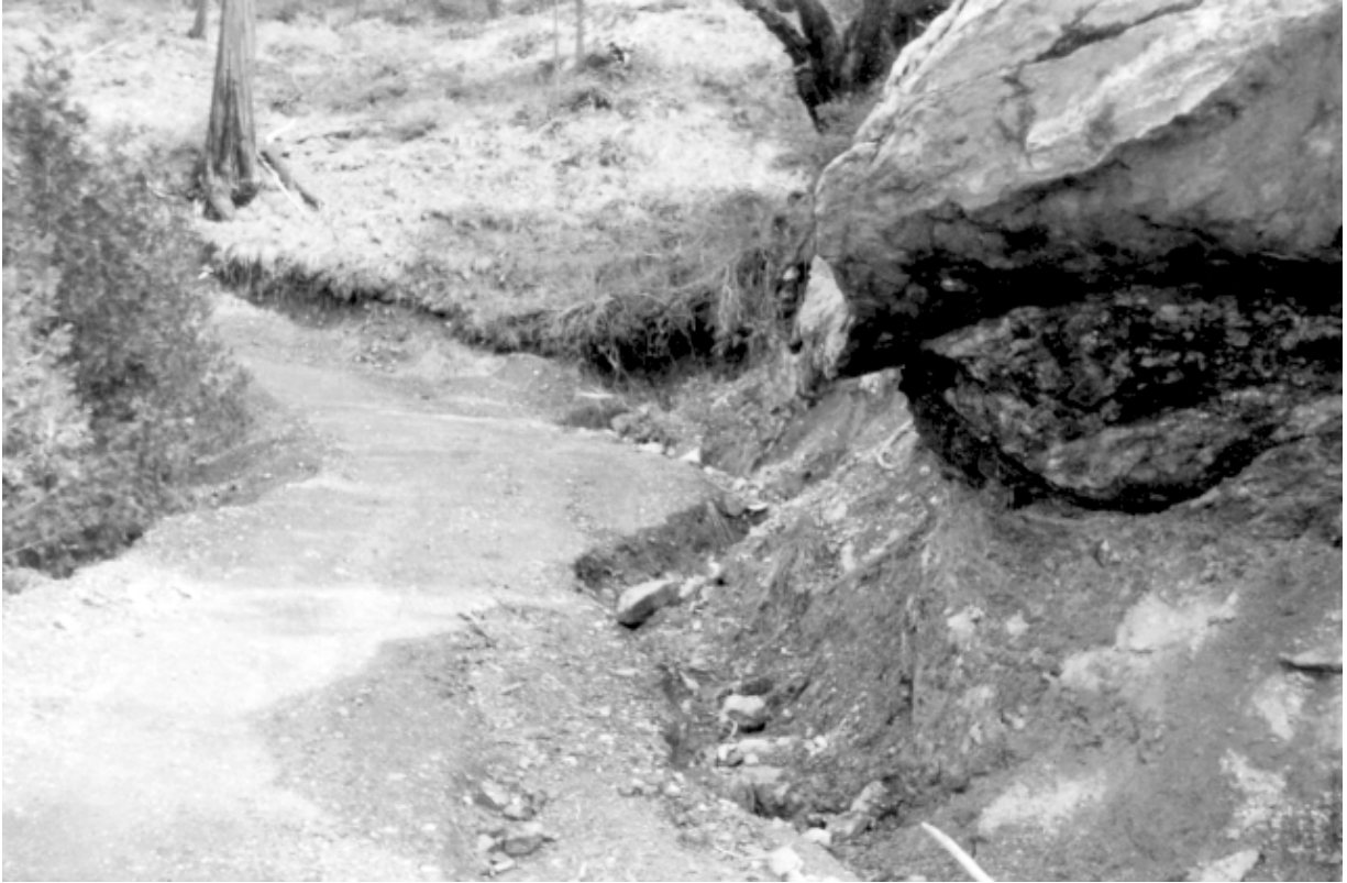
Figure 5—Enlargement of a roadside ditch as a result of stream diversion. The receiving channel (not pictured) has received both sediment and additional runoff as a result of stream diversion.
