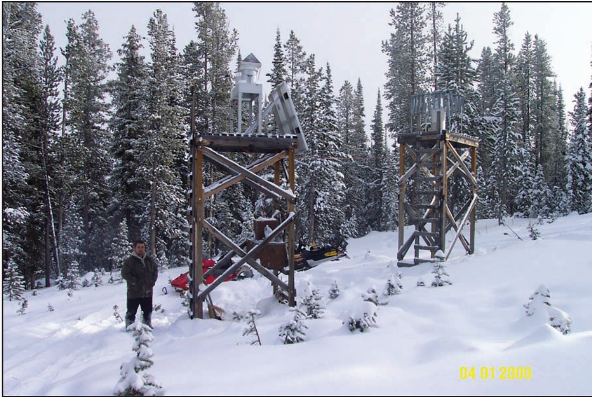
Figure 12—Lost Trail pass (MT97) NADP Site.
