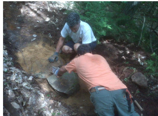
Volunteers install rock armouring. WMNF photo.
