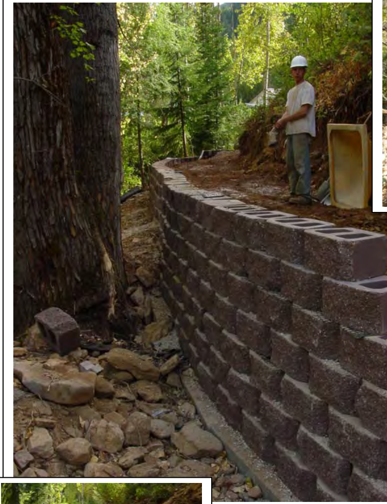
Various stages of modular block wall construction, including installation of the wall drain system.
