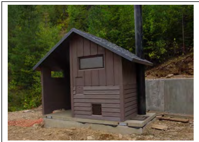
The upper section of the toilet was re-set but sustained damage in the manufacturer's plant and was not accept. The entire toilet is schedule to be replaced.
