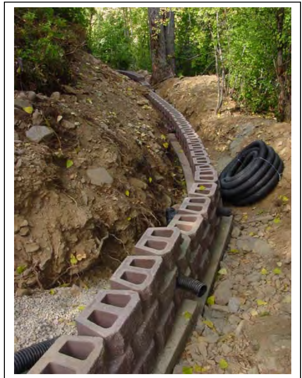
Various stages of modular block wall construction, including installation of the wall drain system.
