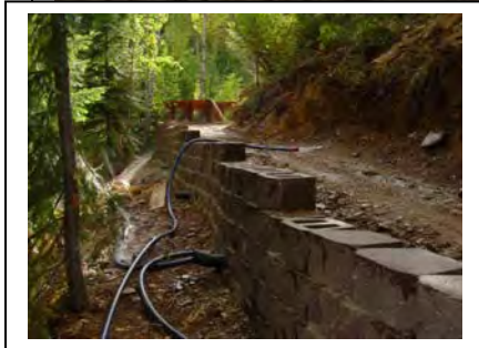
Various stages of modular block wall construction, including installation of the wall drain system.
