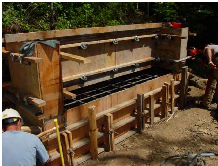
WORKERS FORMING ABUTMENT NO. 2
