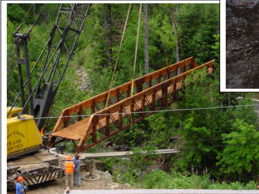
Setting the prefabricated Moosman Bridge on cast-in-place abutments.
