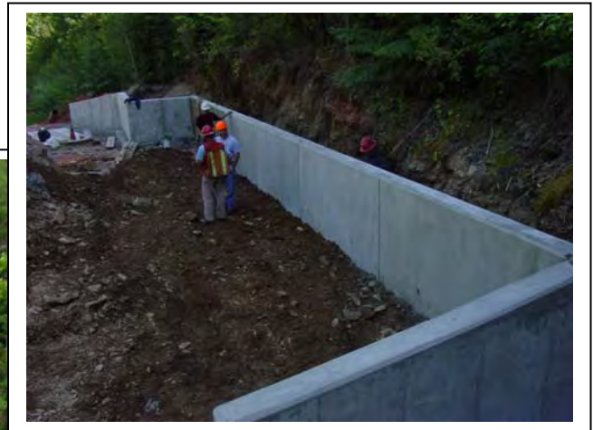
Construction of the parking area concrete retaining wall.
