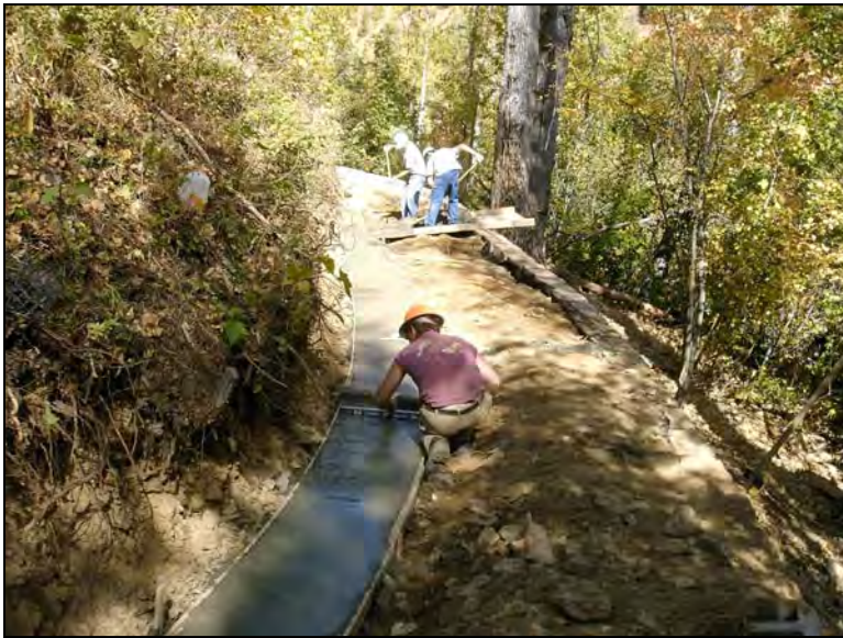
Workers placing concrete for upper modular block retaining wall footing.
