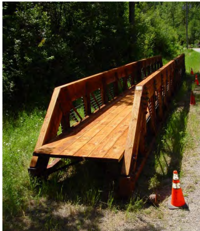
MOOSMAN BRIDGE STOCKPILED ON SITE
