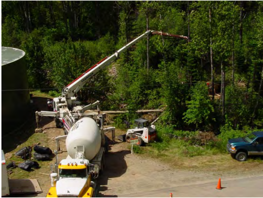
CONCRETE BEING PUMPED FOR ABUTMENT NO. 2
