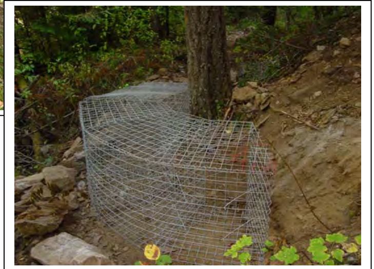
Partially completed gabion basket section at the base of switchback
