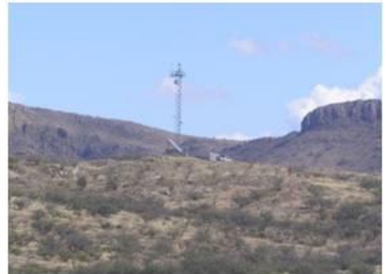
The linear shape of this border surveillance tower contrasts with the rugged and irregular landforms.
