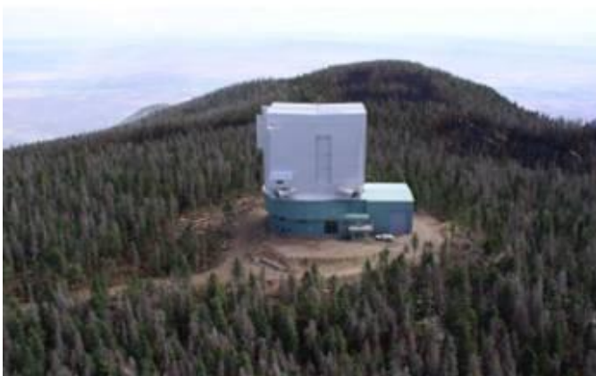
The boxy shape, light color, and scale of the Mt. Graham International Observatory dominate the setting in this conifer forest. Normally the ESI for something like this would be Unacceptably Low, but the visual quality objective for this area was modified by amending the forest plan.
