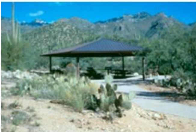
The Cactus Environmental Education Ramada provides needed shade while using colors from the mountains, and has Moderate Scenic Integrity.
