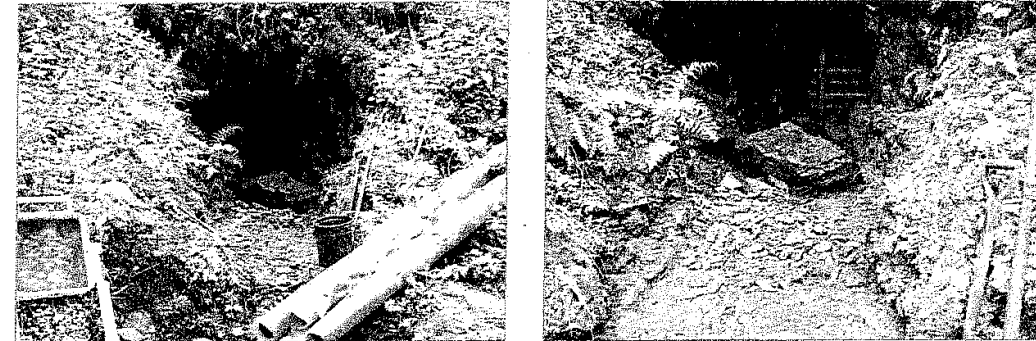
Figure 6. Prior to setting the posts and caps Forest Archaeologist, Steve Matz, systematically removed the material from in front of the portal with a trowel looking for artifacts. Since the material was so wet and rocky it couldn't be screened, but had to be removed very carefully so that any pieces of horse tack or other artifacts associated with the Pulaski crew could be found. All fill material in the area of the posts was removed by trowel down to where clean, undisturbed rock was found. Once troweled the fill was placed back into the mouth of the portal near the metal gate. While only three pieces of heavy sheet metal were found in the fill, contractor Dwight Clift said he had seen decayed pieces of horse tack in the area only several years before.
