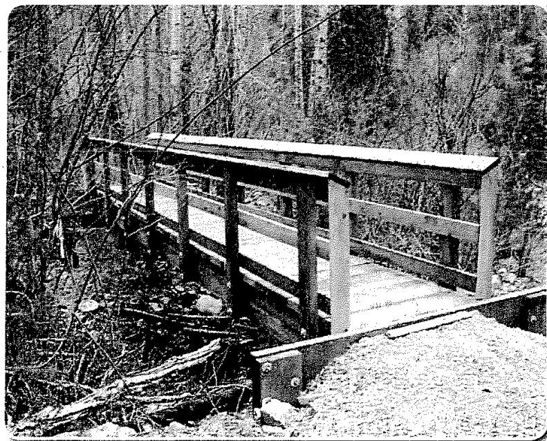
Treated Timber Bridge, No. 1
