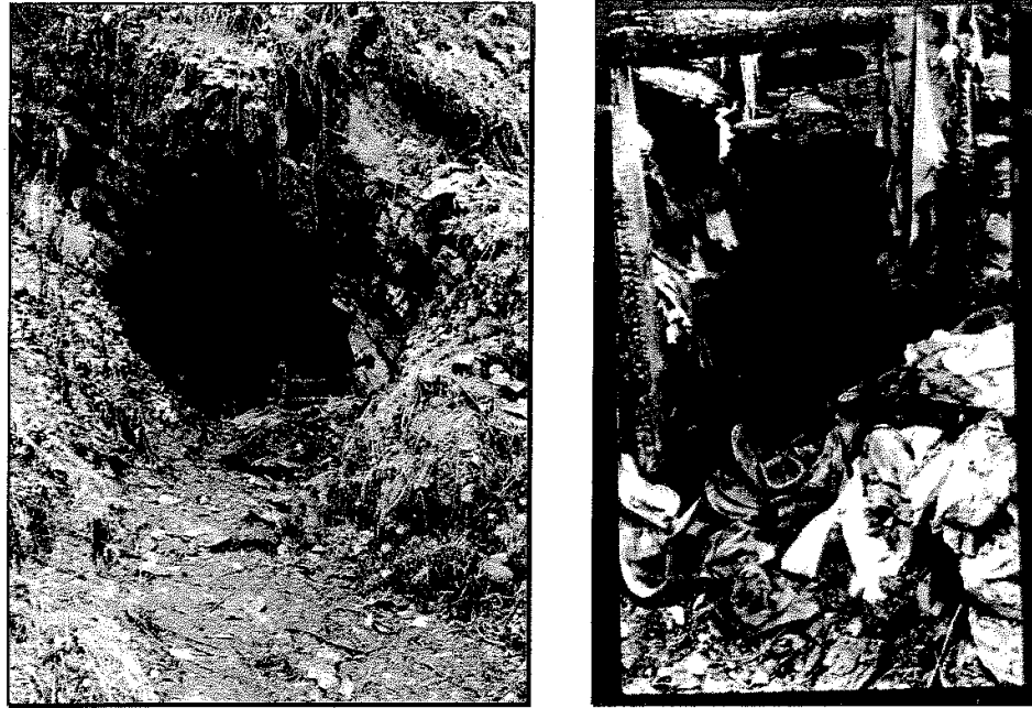
Figure 7. Present adit with gate installed (left) and original 1910 portal with saddles and other material at entrance immediately after fire (right).
