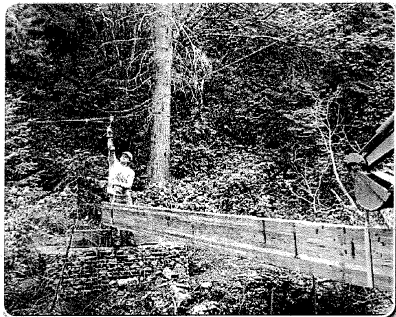
Setting the 1st Glu-Laminated Stringer with hand cable assembly
