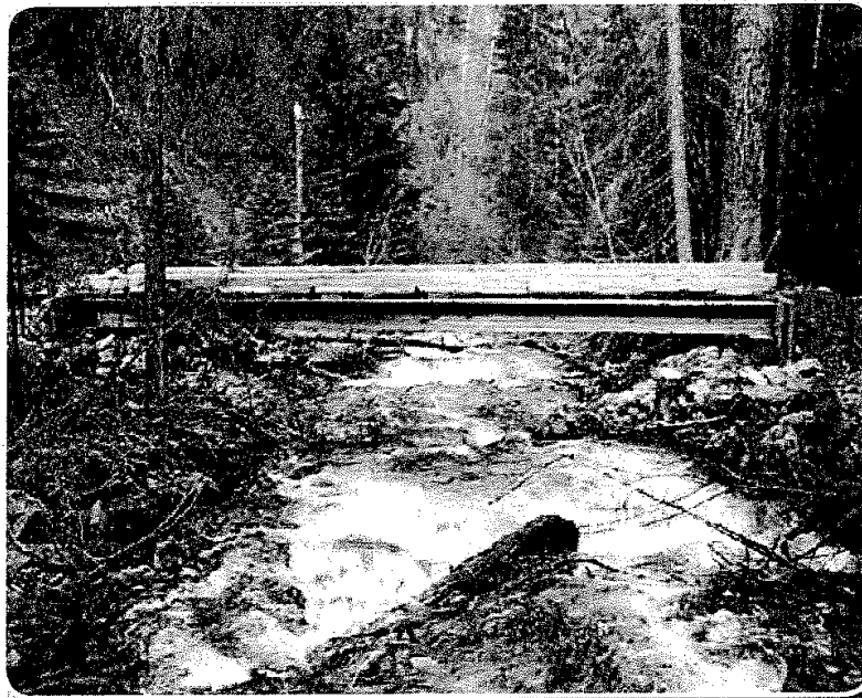
Treated Timber Trail Bridge No. 2, West Fork Placer Creek.
