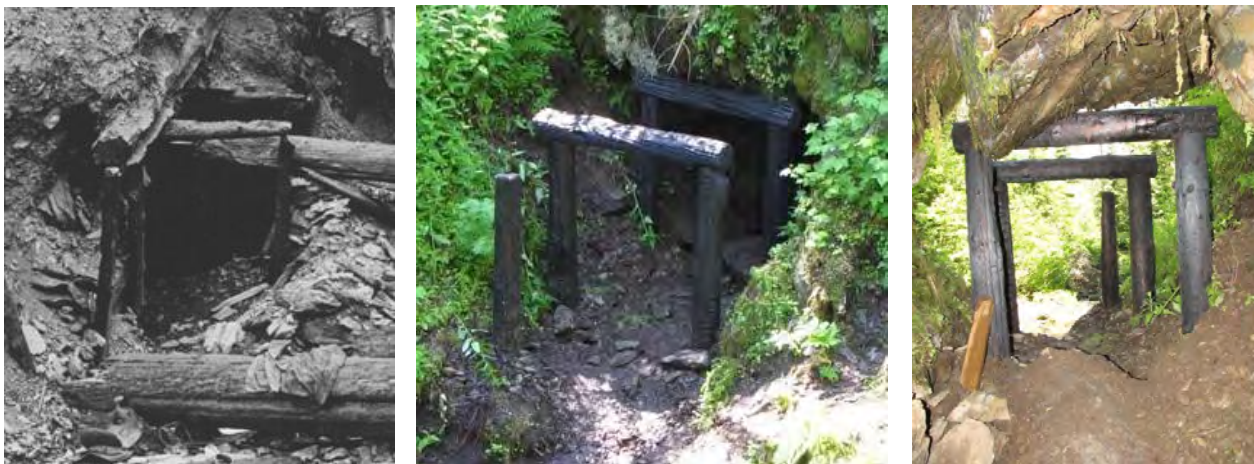
Figure 4. Pulaski Tunnel Portal reconstruction. Post 1910 photo (left), post restoration outside (middle), and post restoration inside (right).
