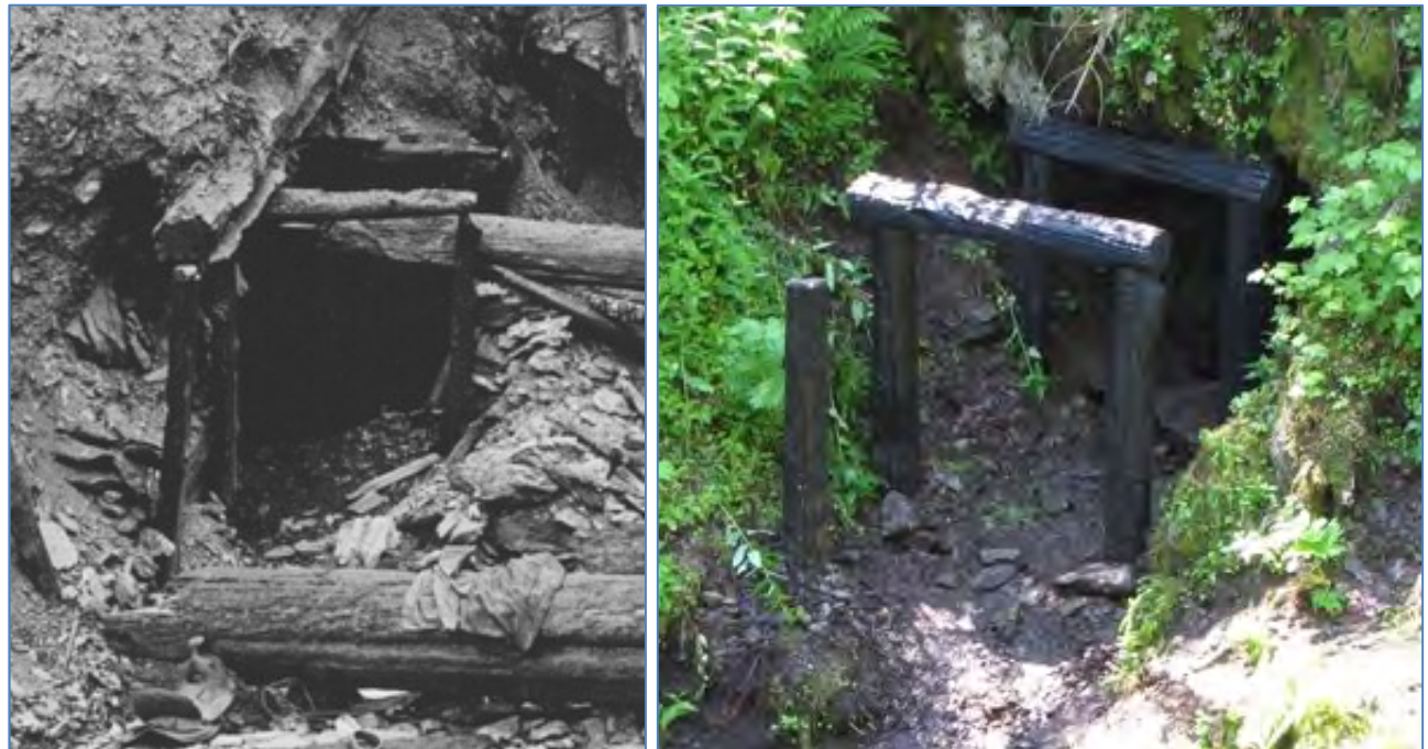
Figure 11. Enlargement of portal section of 1910 McKay photo on left showing original post fire condition and post reconstruction photo taken upon completion of project in 2010 on right.
