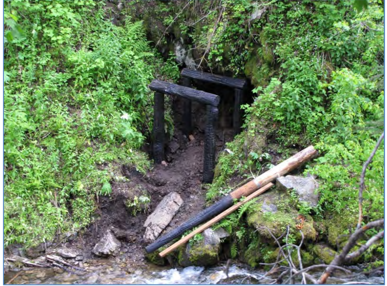
Figure 8. Dwight and Steele level posts in order to set cap log in the left photo, while the right photo shows the two sets nearly finished and the uncut final post lying on the ground.
