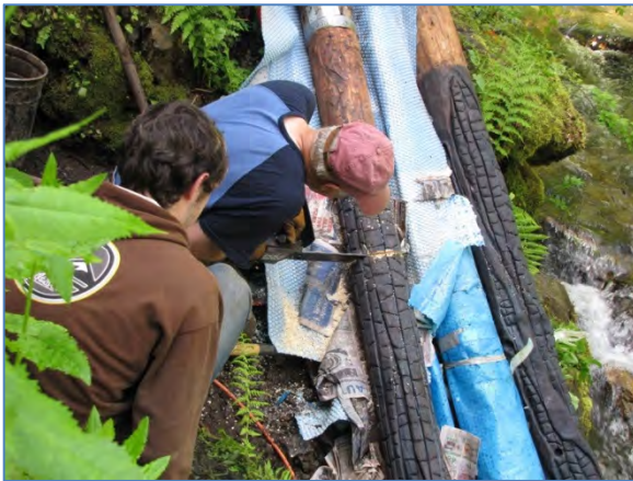
Figure 4. Intial construction of the adit portal sets. Dwight Clift and grandson Steele cut the posts to length with an electric chainsaw (left photo), while Steele steadied the post for Dwight to nail brace into place (right photo).
