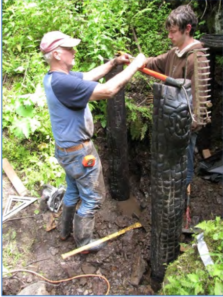
Figure 8. Dwight and Steele level posts in order to set cap log in the left photo, while the right photo shows the two sets nearly finished and the uncut final post lying on the ground.
