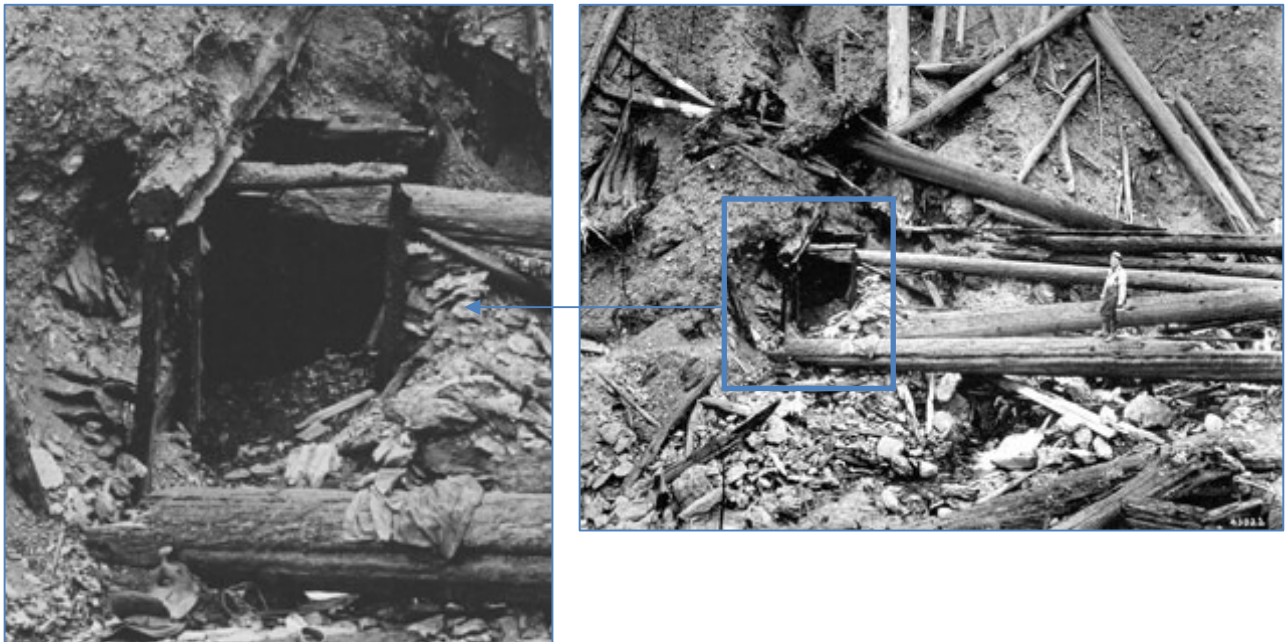
Figure 1. Post fire photograph of W.W. Morris by R.H. McKay of the Nicholson Adit on right and enlarged view of adit portal from same photo on left (photo courtesy of Northern Region Forest Service Archives).
