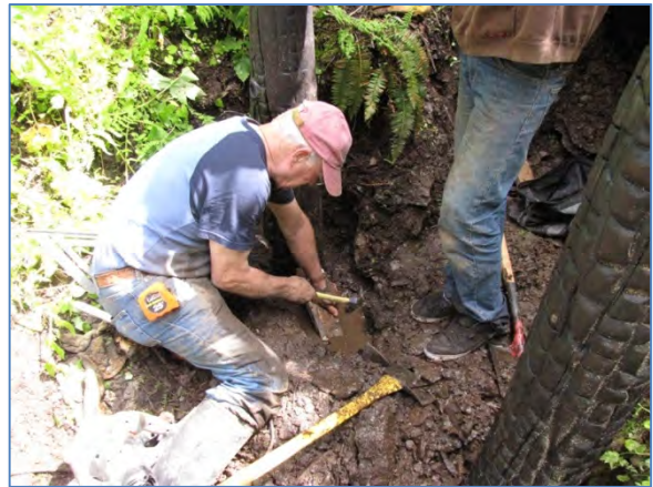
Figure 4. Intial construction of the adit portal sets. Dwight Clift and grandson Steele cut the posts to length with an electric chainsaw (left photo), while Steele steadied the post for Dwight to nail brace into place (right photo).
