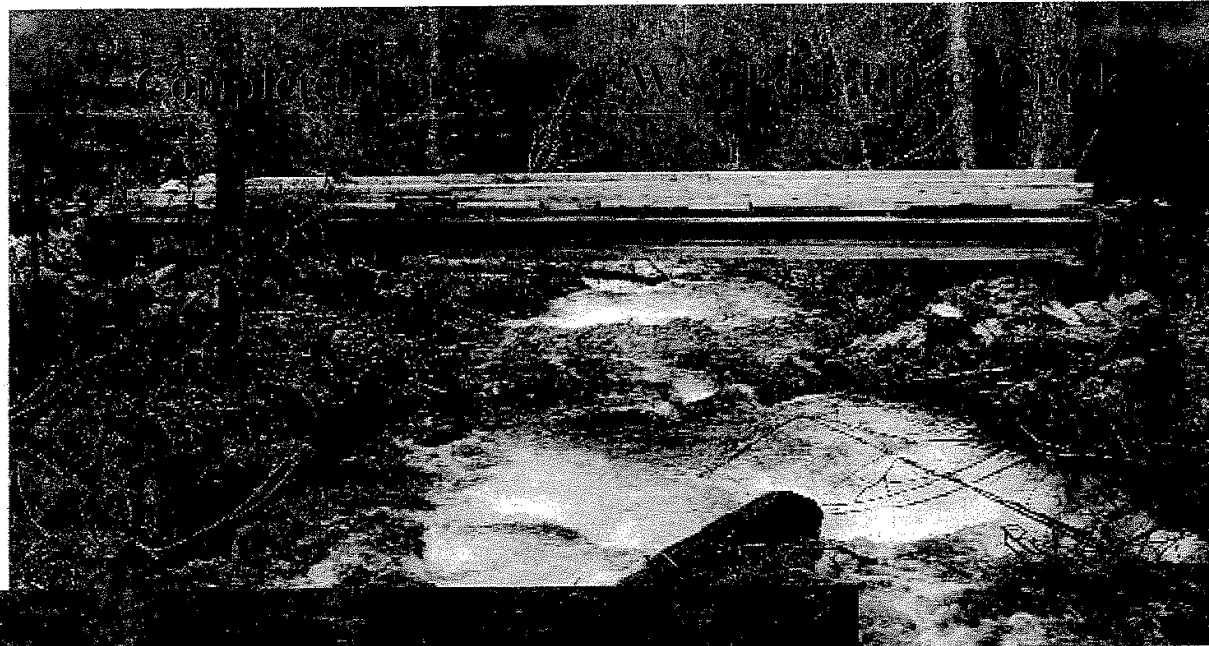
Final 24 Foot Span Foot Bridge Installation Over Tributary to West Fork Placer Creek
