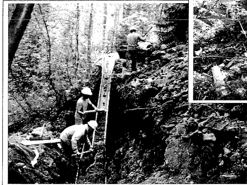
Workers placing concrete for block wall footing. Upper picture is modular block wall nearing completion at same location.
