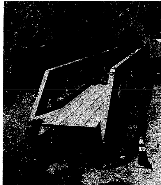
MOOSMAN BRIDGE STOCKPILED ON SITE
