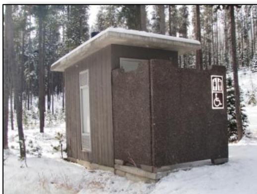
New privacy screens on a Many Pines Campground vault toilet.
