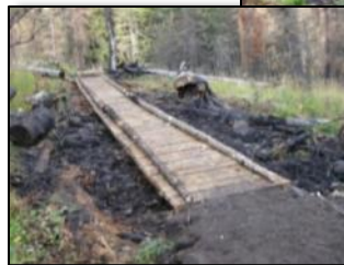
A mudhole on the Hellroaring Trail before and after puncheon construction.
