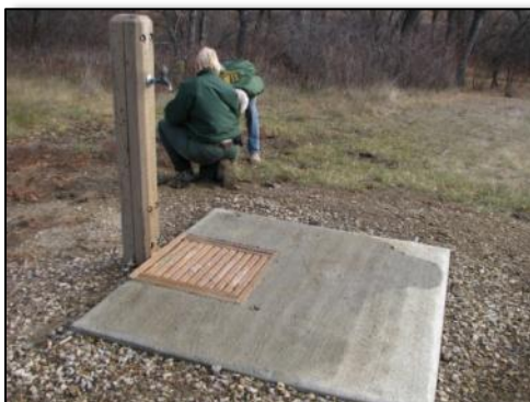
New water hydrant at Buffalo Gap
