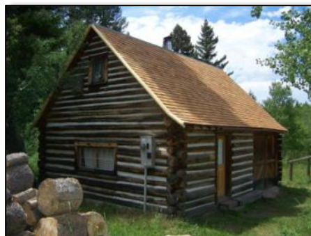
Bear Creek Bunkhouse's new roof
