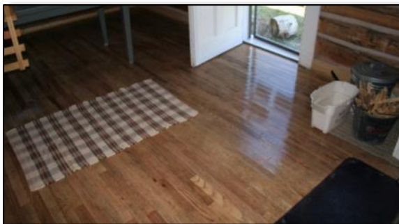
Refinished floor at Black Butte Cabin
