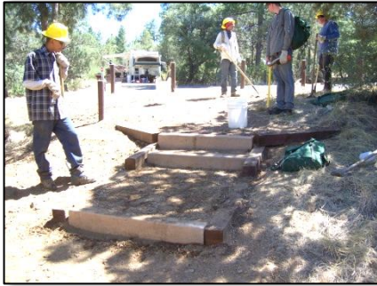
YCC crew repair stairs at Hilltop Campground.
