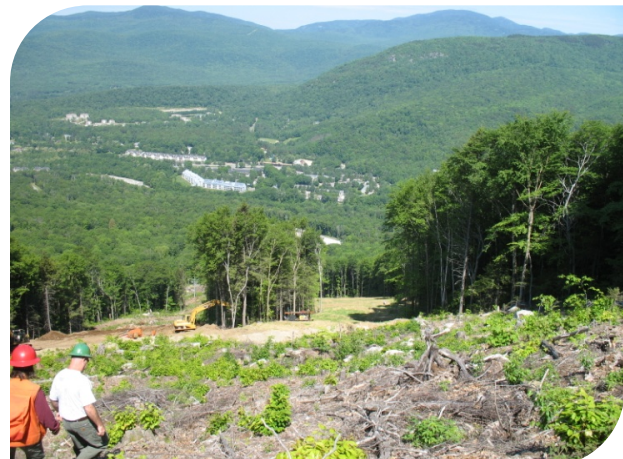
Straw mulch, grass and water bars to prevent erosion on trails 41&42 South Peak, Loon Mountain. WMNF photo by Andy Colter.
