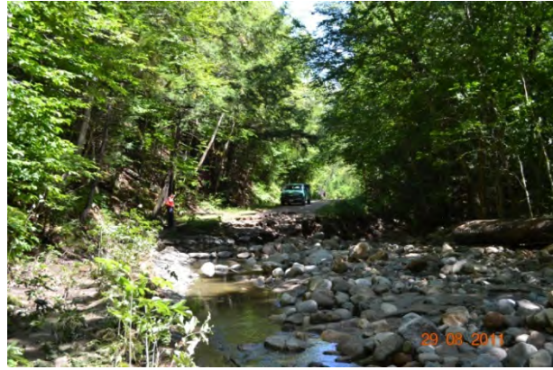
Tunnel Brook Road after the brook was back in its banks. WMNF photo by Chris Mattrick.
