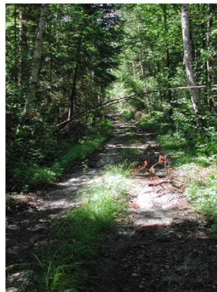
Unauthorized road. WMNF photo by Kori Marchowsky
