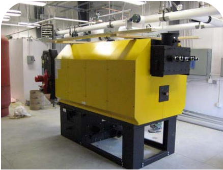
Biomass boiler at WMNF Headquarters building. WMNF photo by Bill Dauer.
