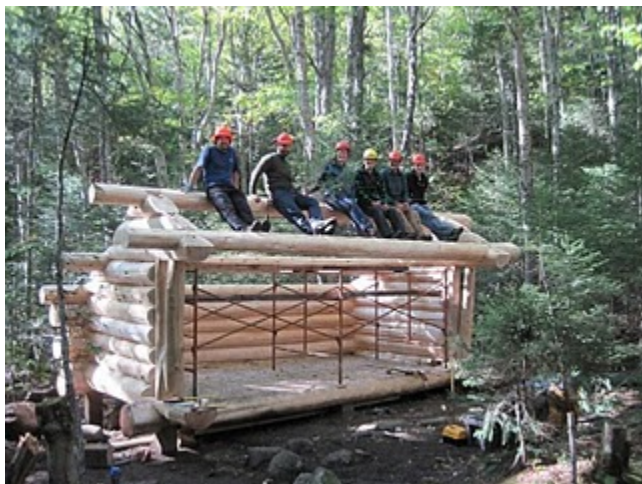
Replacing the Eliza Brook Shelter. AMC photo.
