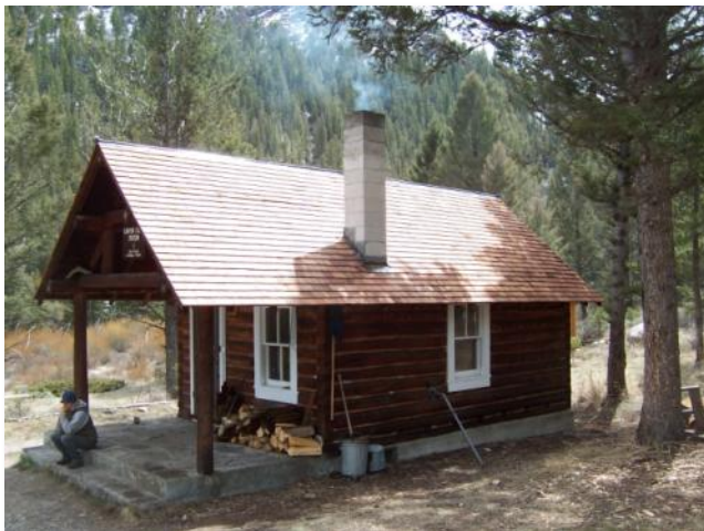
Workers installing a new shake roof at Moose Lake Cabin.
