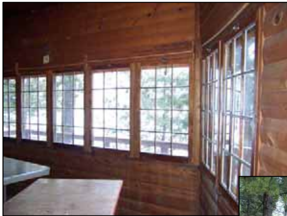
Repaired and reglazed windows at Woods Cabin
