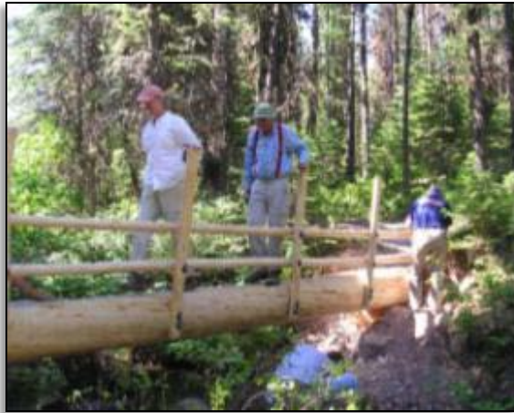
A log footbridge under construction on the Clearwater Lake Trail
