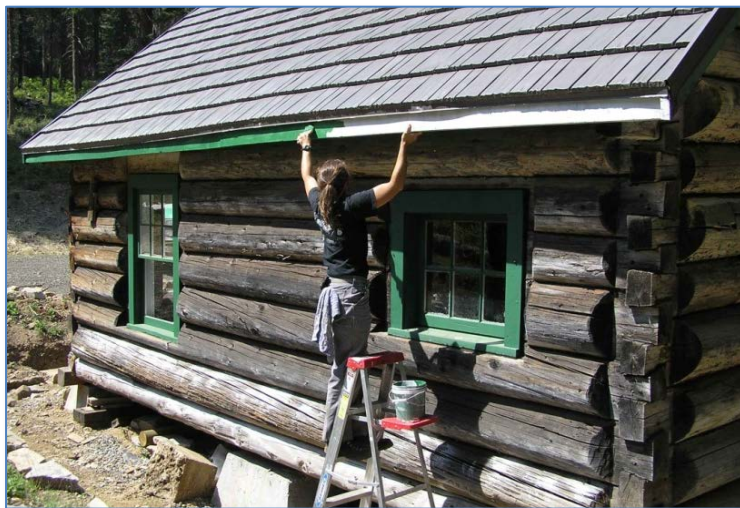
Adams Camp repairs and restoration work
