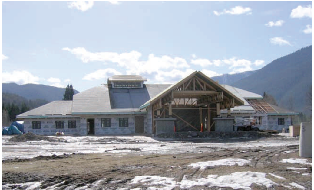
Construction is underway on the new Hungry Horse/Glacier View office.
