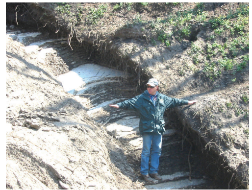
Gates of the Wilderness washout & erosion after fires.
