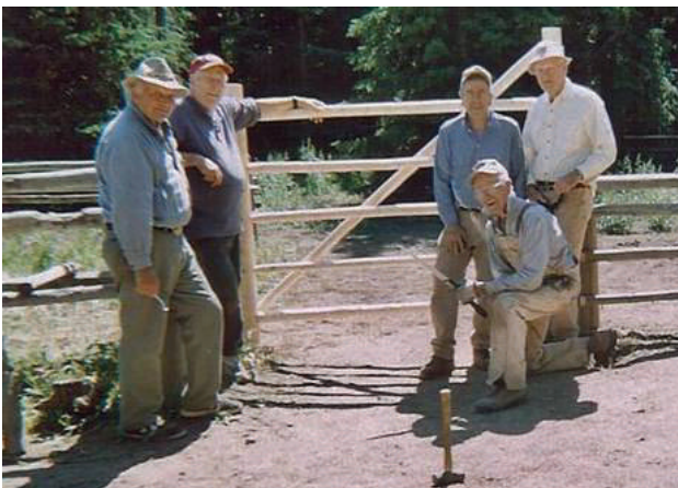
NSA crew replacing a gate at Webb Lake Guard Station.
