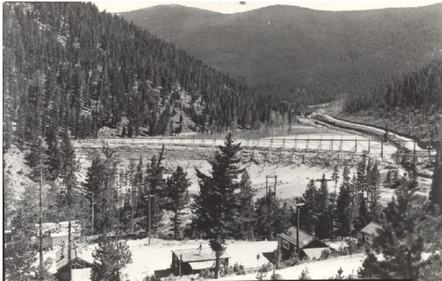
MIKE HORSE DAM DURING CONSTRUCTION (CIRCA LATE 1940'S)
