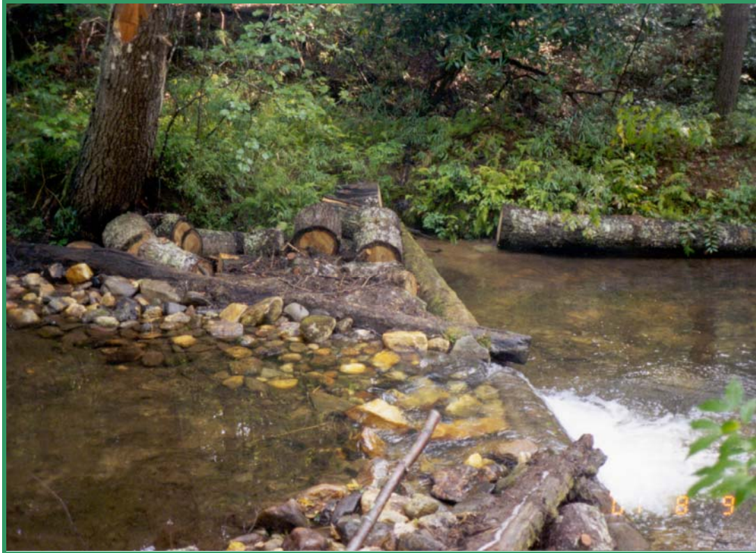
Figure 18 – Repairs completed on a K-dam structure over thirty years old
