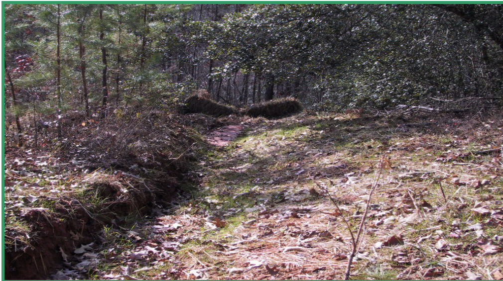
Figure 17 - New Wing-Ditch with Hay Bales (Background) Installed to Catch Silt
