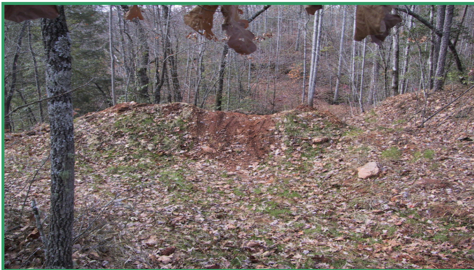
Figure 14 - Blocked Temporary Use Road That Has Been Breached
