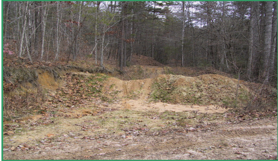
Figure 15 - Side Roads Blocked and Breached
