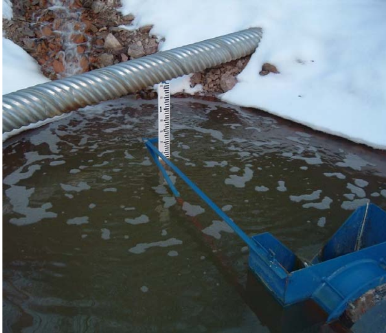
Figure 6.5 Weirs can be constructed to measure flow at all major water quality monitoring locations.
