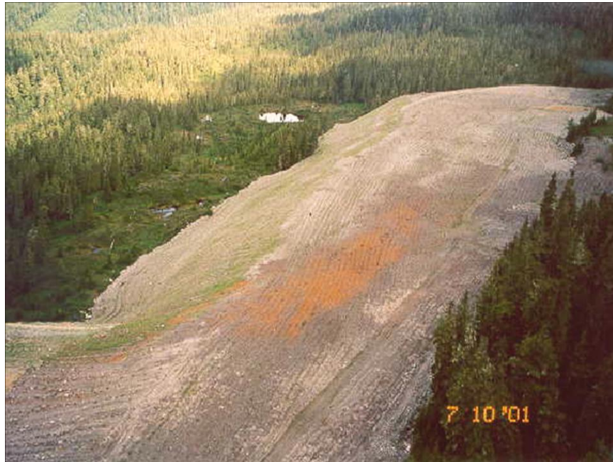
Figure 3.8 There is significant uncertainty regarding some aspects of drainage chemistry at most major precious and base metal mines and many coal mines in Canada (photo of Kitsault Mine in northwest British Columbia).
