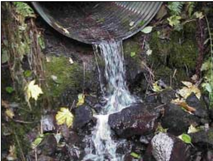
Figure 42. Metal culvert barrier to southern torrent salamanders on Thunder Creek.
