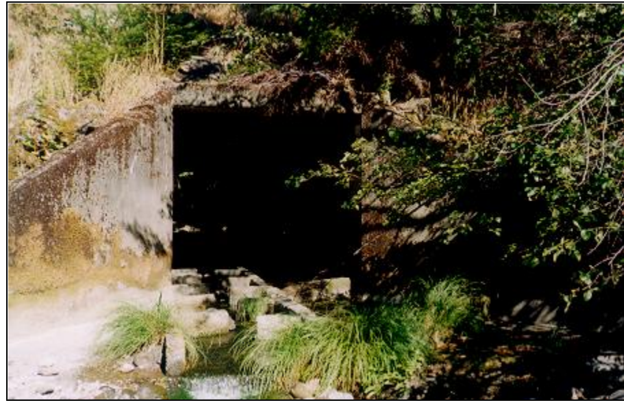
Figure 39. Cement culvert, with a fish passage structure, at the mouth of Williams Creek.
