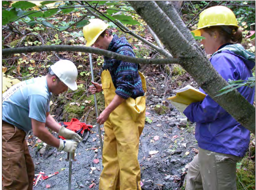
Engineers Ben Dreier, Pete Bolander, and Amy Klein set up a drive probe to determine the distribution and estimated strength of subsurface soil units.
