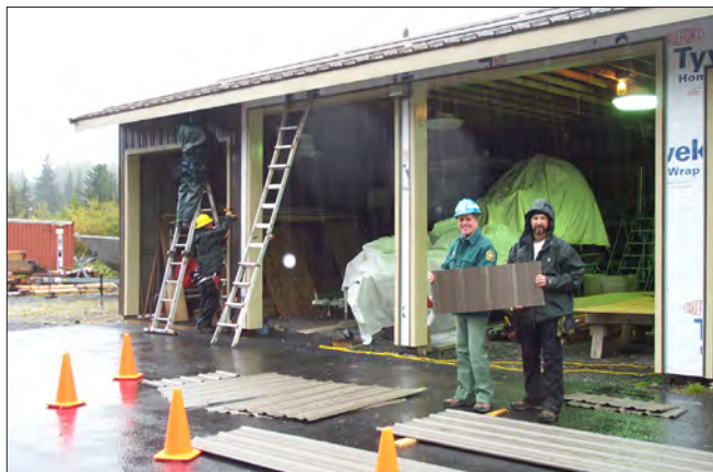
New pole barn and warehouse in Cordova.
