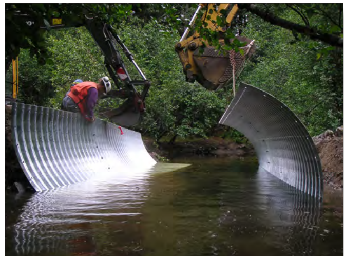
Peter Cross works on a replacement arch culvert.
