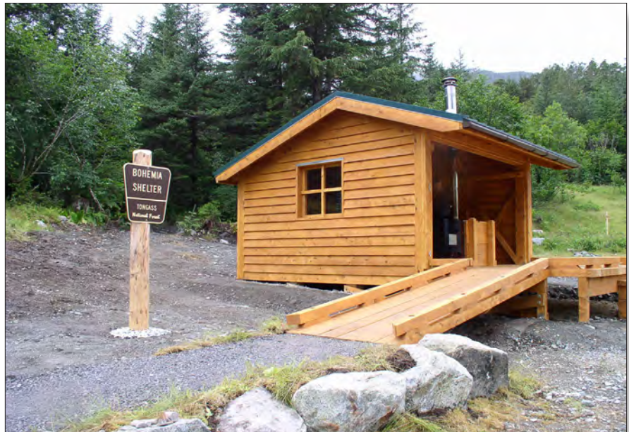
Tongass wood was used in the construction of this emergency shelter at Bohemia near Pelican. Photo by Forest Service Recreation staff.
