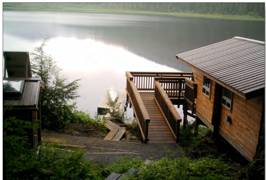
The approach to the popular Windfall Lake Cabin has been converted to make the cabin more accessible. Photo by Rob Morgenthaller.
