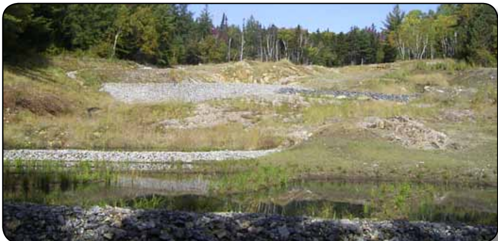
Figure 22. Tailings area of Ore Hill site with constructed wetlands in foreground to provide passive treatment. WMNF photo by Sheela Johnson.
