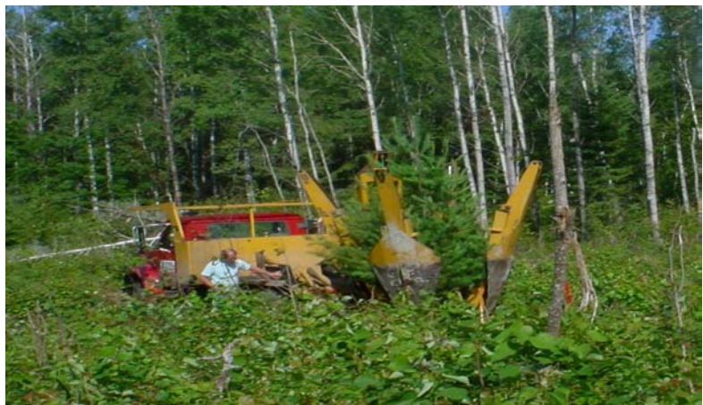
Tree spading white pine into openings in an aspen stand.
