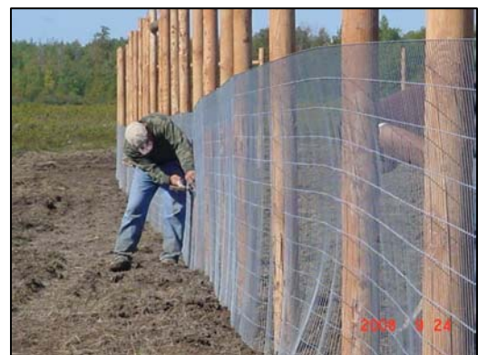
Constructing the deer enclosure at the planting sites.
