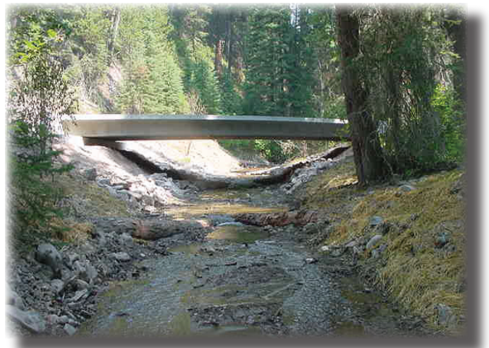
Lolo National Forest culvert - after replacement
