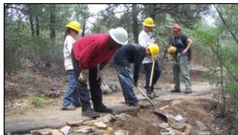
YCC crew improving drainage structures on Trail 311.
