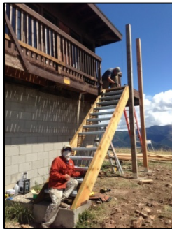
Garnet Mountain Lookout gets a new staircase and catwalk.
