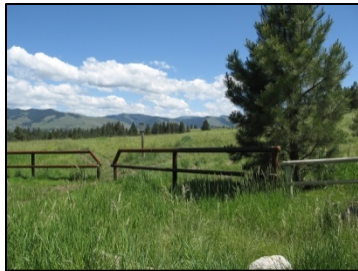
Steel fence constructed from repurposed drill steel at Blue Mountain recreation area.
