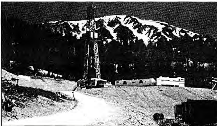
SEVERAL EXPLORATORY WELLS HAVE BEEN DRILLED ON THE NORTHERN PORTION OF THE NATIONAL FOREST
