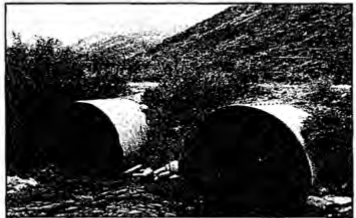
Culverts reduce stream sediments from roads
