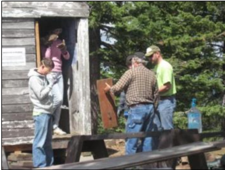
Partners assist with the renovation of Spyglass Lookout Round House.
