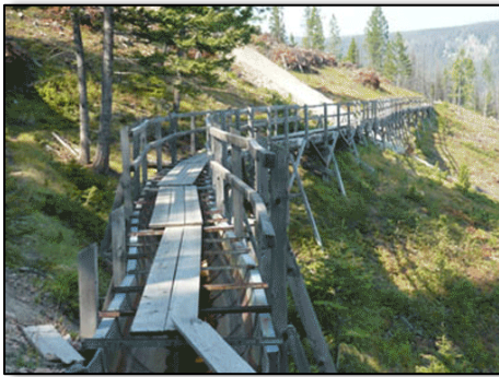
Red Mountain Flume Chessman Reservoir
