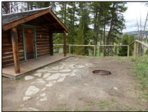
The Wapiti Cabin got a new porch floor, patio and fire ring.
