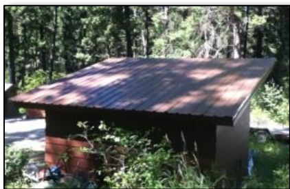
Warm Springs pump house's new roof
