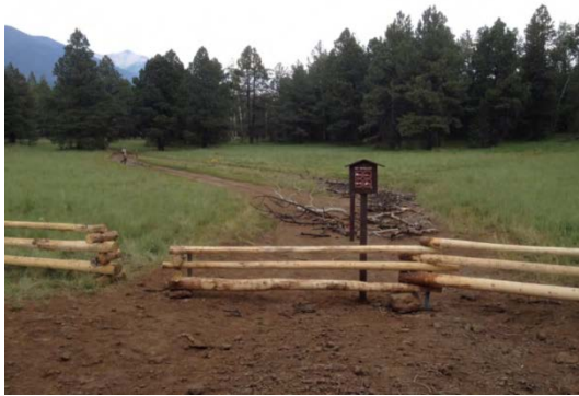
Figure 10. Completed log fence blocking vehicular access to unauthorized road through meadow area
