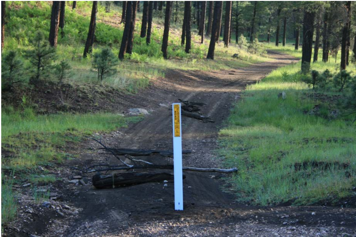
Figure 3. Carsonite sign installed on non-designated road to prevent unauthorized motor vehicle use
