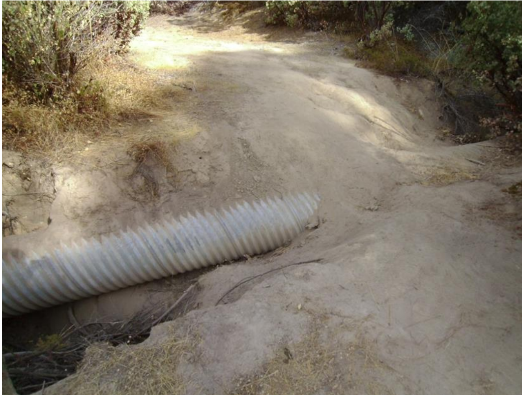
Figure 5: Exposed culvert on Forest Road 13S97B
