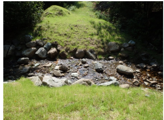
Higgins Brook site after restoration. WMNF photo by Jay Milot.
