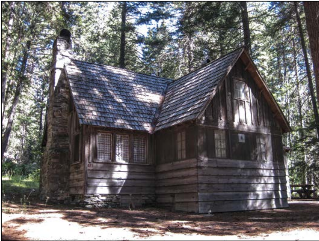
Figure 23—The foundation of this 1938 recreation residence at the Indian Creek tract of the Okanogan-Wenatchee National Forest in the Pacific Northwest Region raises the floor 1 to 3 feet above the gently sloping ground.
