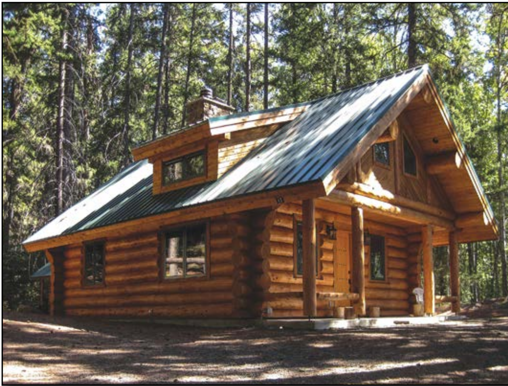
Figure 35—This replacement recreation residence at the Okanogan-Wenatchee National Forest’s Indian Creek tract in the Pacific Northwest Region was built in 2006. The size, general shape, proportions, window-to-wall ratio, colors, and materials are reasonably similar to historic residences in the tract, but the design doesn’t mimic the historic buildings.
