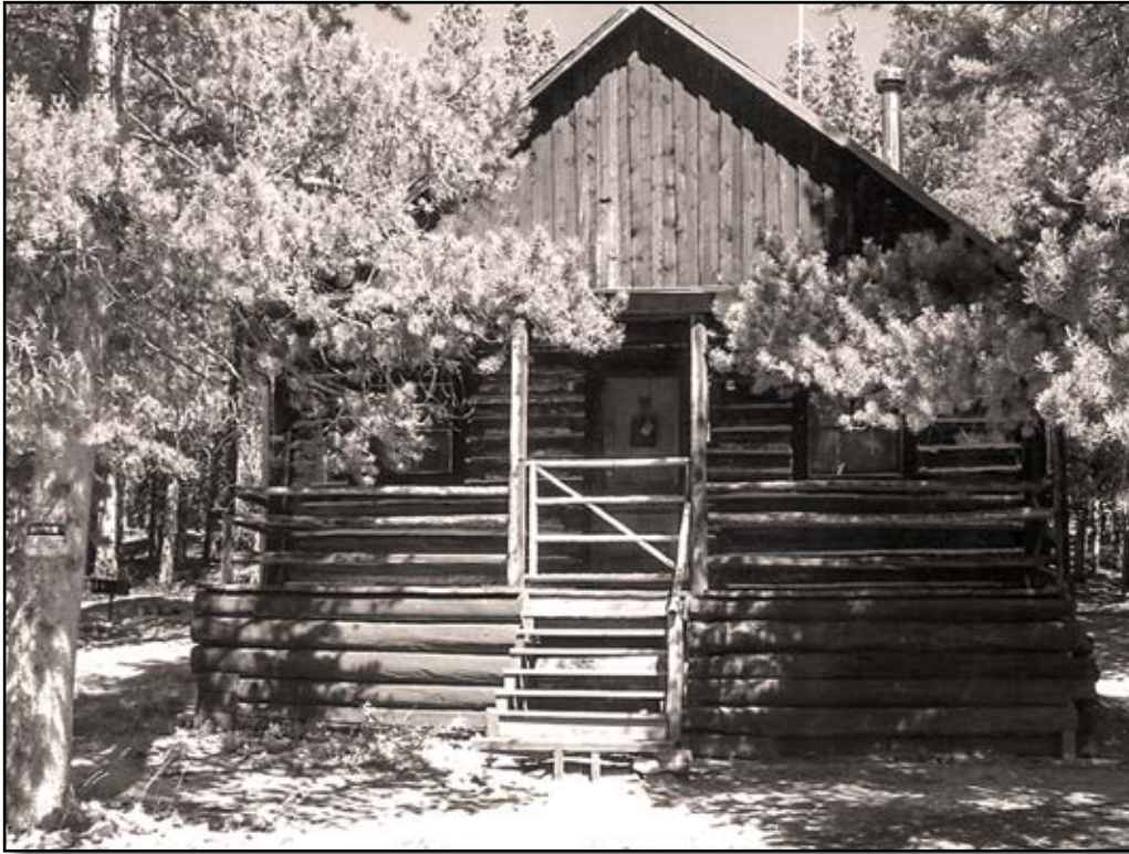
Figure 13—The peeled log porch posts and rails add a rustic appearance to this recreation residence, which is part of the Gramm tract of the Medicine Bow-Routt National Forest in the Rocky Mountain Region. The 1905 cabin, the oldest cabin at the Gramm tract, once served as a general store.
