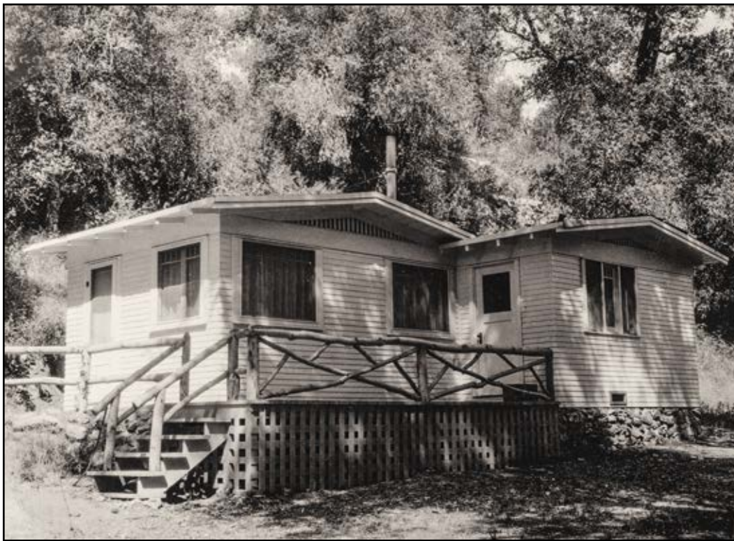
Figure 2—This recreation residence in a riparian canyon of the Cleveland National Forest in the Pacific Southwest Region has character-defining features typical of that area in the 1920s: a distinctive low-slope roof with exposed rafter tails, rock foundation, narrow beveled lap siding, rustic pole railings, perpendicular lattice under the porch, and removable screens on each window.
