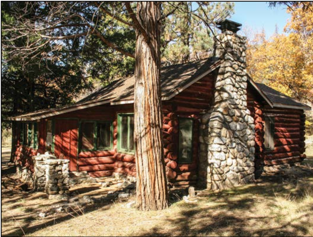
Figure 30—Located at the Seven Oaks tract of the San Bernardino National Forest in the Pacific Southwest Region, the addition on the back of this log recreation residence is compatible in size and construction.
