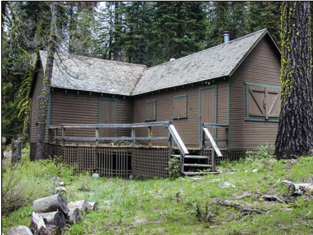
Figure 4—The snow shutters have not yet been removed for the summer from this recreation residence high in the Sierra Nevada Mountains of the Eldorado National Forest in the Pacific Southwest Region.
