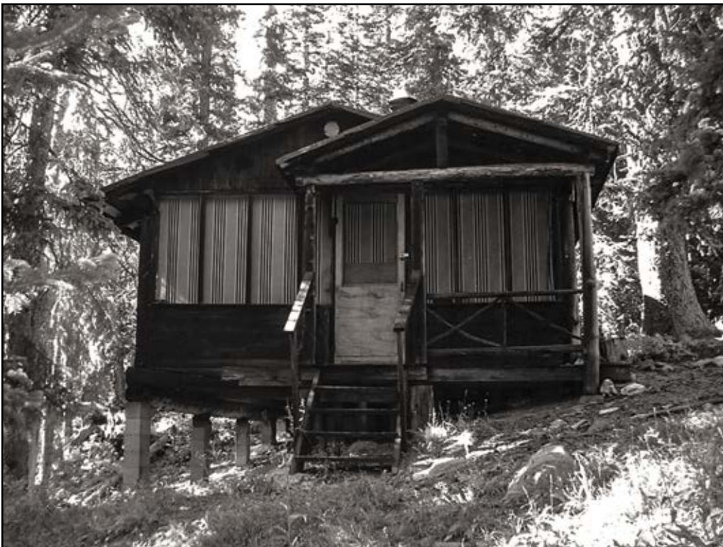
Figure 24—This recreation residence at the Cascades tract of the Medicine Bow National Forest in the Rocky Mountain Region was built in 1927 on a concrete block post and beam foundation—a relatively inexpensive method to support a building on a sloping lot. This foundation may not meet current building codes.
