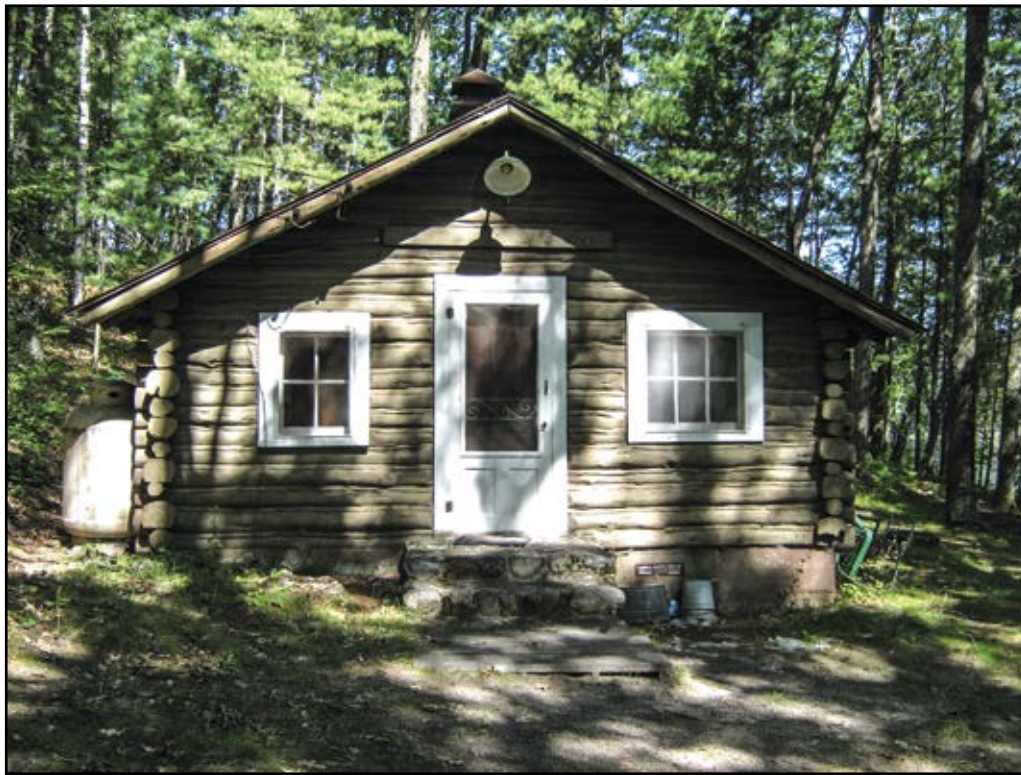
Figure 21—The wood screen door is original to this small 1938 recreation residence at the Loon Lake tract of the Huron-Manistee National Forest in the Eastern Region.
