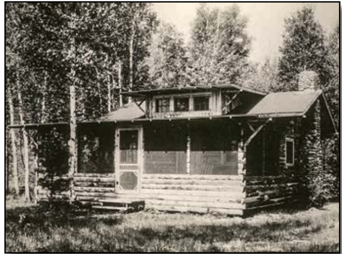
Figure 9—This 1934 photo of a recreation residence at the Deer Lake tract of the Chequamegon-Nicolet National Forest in the Eastern Region shows a shed-type dormer with windows that bring extra light to the interior of the building. The original photo caption: “Very good type of summer home construction.”
